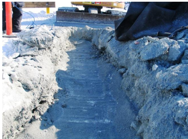
Photo 6: Bedding for cables...core material
