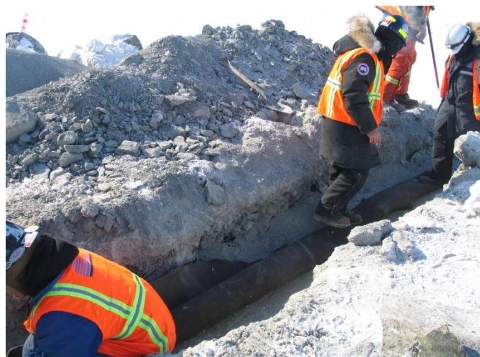
Photo 8: Wrapping cable with geotextile.
