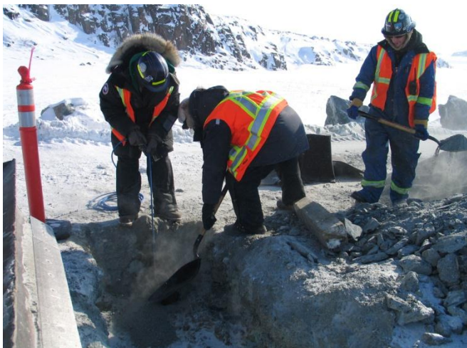
Photo 7: Backfilling hole.
