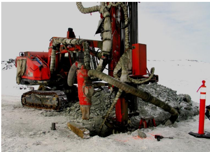
Photo 5: Drilling for thermister SRK –DWB5
