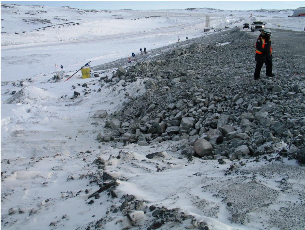
Photo 2: Downstream slope between Sta 0+20 and 0+40 still needs to be graded and packed.
