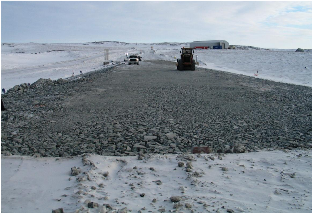
Photo 1: Progress photo of North Dam facing north. Photo shows ROQ placed April 6 th . 10 ton packer is starting to pack.
